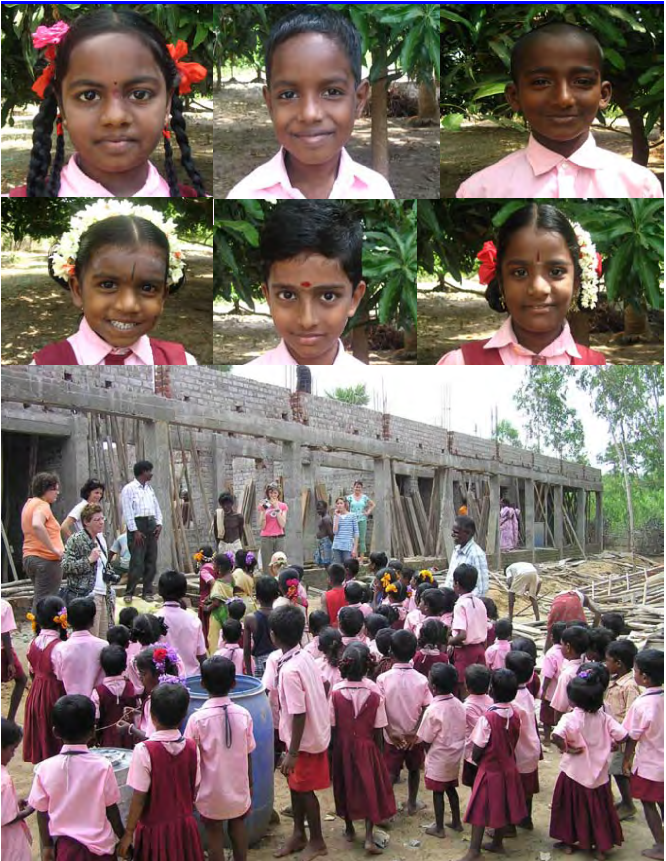
The Mother Teresa School children come to admire the ongoing construction of their new school, which is expected to be inaugurated at the start of the next school year in June 2008.
